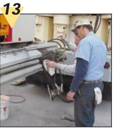
Remove the feeder drive motor from the collet and let it hang by the hoses. Remove the collet and clean the collet bore. Inspect the collet splines, drive motor splines, collet key and collet keyway for wear. Replace worn parts upon reassembly.
