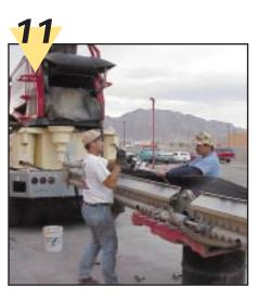
Remove the u-rollers, upper side idler rollers, discharge boot and head scraper assembly. It is not necessary to remove the bottom rollers.
