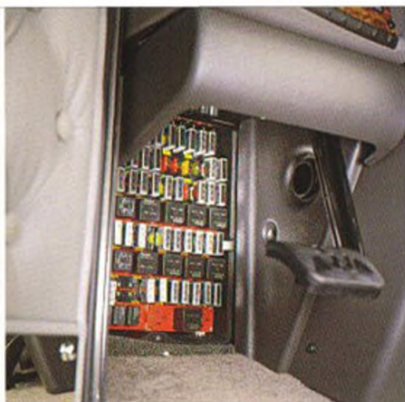
The W900's power distribution box puts all circuit protection elements – fuses, relays and breakers – in one quick-to-reach location.
