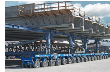
BRIDGE & TUNNEL CONSTRUCTION
