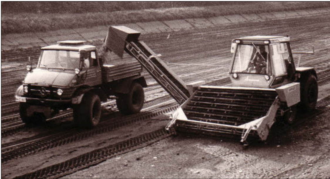
Doppstadt cleaner for filter basin cleaning, first self-propelled machine
