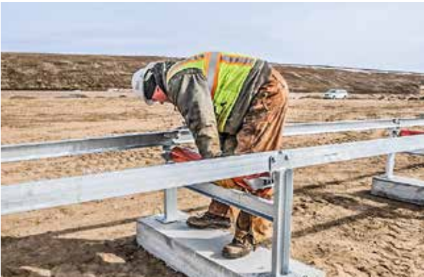
INTEGRATED RETURN IDLER BRACKETS
