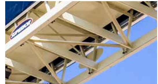
C/ STINGER CROSS BRACING
