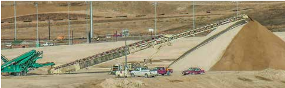
LOW PROFILE ELIMINATES TRANSFER CONVEYOR BETWEEN PLANT AND STACKER
