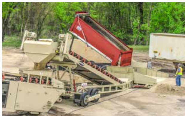
END DUMP TRUCKS TO MATERIAL STOCKPILE
