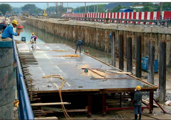
Flutunnel in Kuala Lumpur
