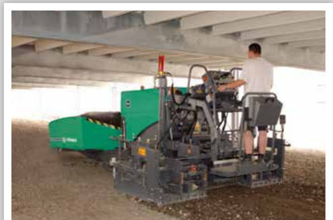
BUILDING THE BASE FOR PAVING SETTS
