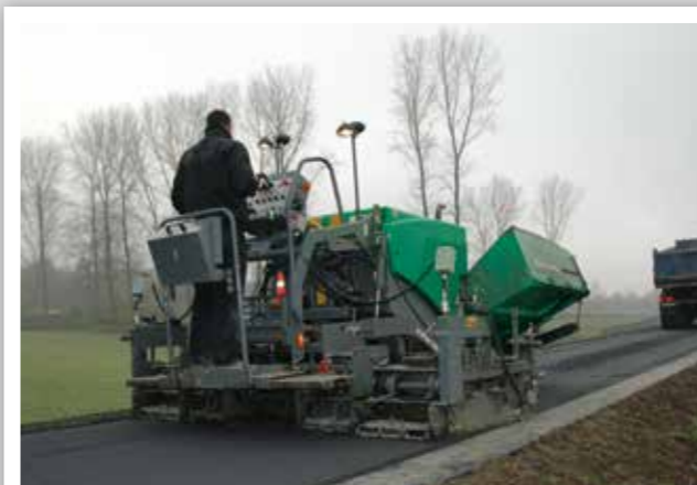
PAVING ASPHALT ON DAMS
