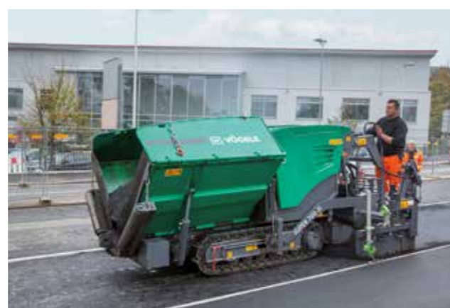
PAVEMENT REHABILITATION ON SMALL MUNICIPAL ROADS
