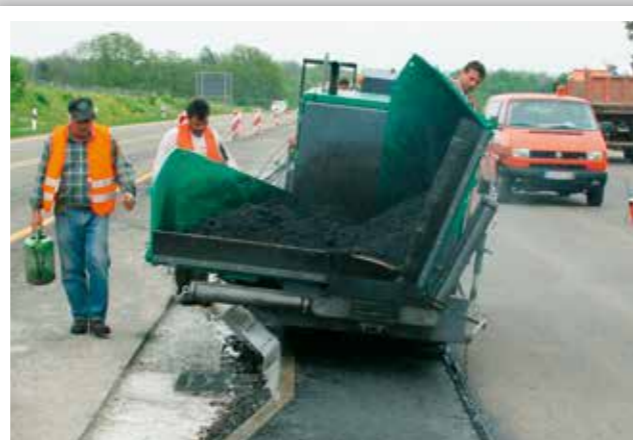
SURFACING MEDIAN STRIPS ON MOTORWAYS
