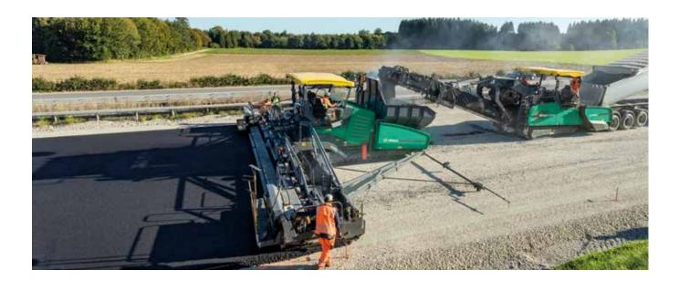
Fixed-width screeds from VÖGELE deliver absolutely high-quality, perfectly even results. They show their strengths wherever large pave widths have to be handled, when laying down thick layers (e.g. crushed-stone bases) and where high degrees of precompaction have to be achieved. The SUPER 3000-3 can be combined with the SB 300 and SB 350 Fixed-Width Screeds.
