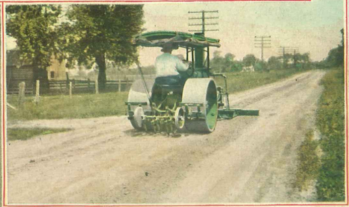
A One-Man Austin Pup making a bad dirt road into a good dirt road at the lowest known cost
