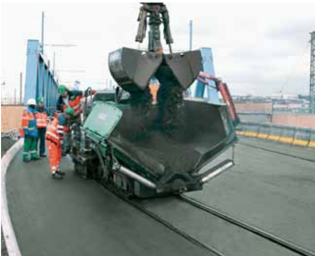
Paving asphalt between tramway tracks
