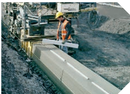
▲ Placing the concrete for a slot drain to ensure storm-water run-off
