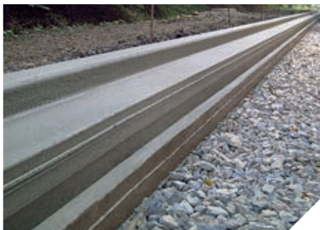
◀ Paving of complex kerb-and-gutter profiles
